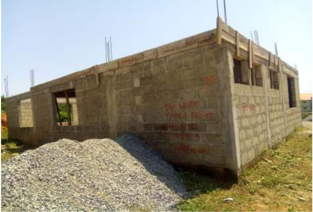
Ryner Paul Anglican School ICT Centre at Roofing Level
