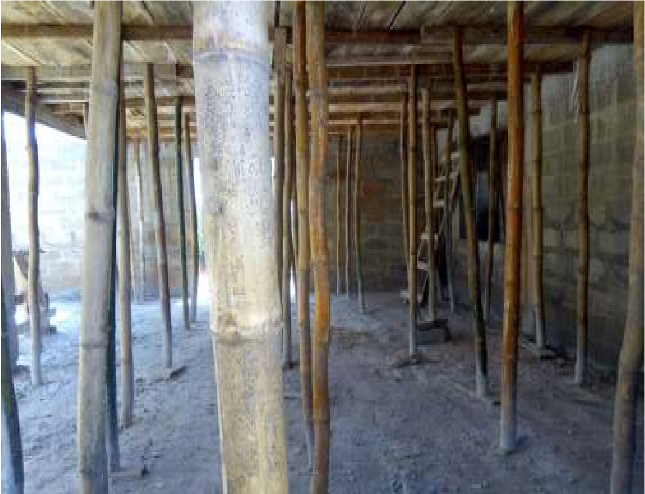
Ryner Paul Anglican School ICT Centre at Roofing Level
